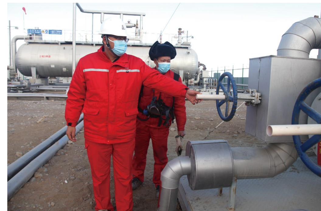
④ Safety management personnel screening for hazards at the Shunbei 5 site
